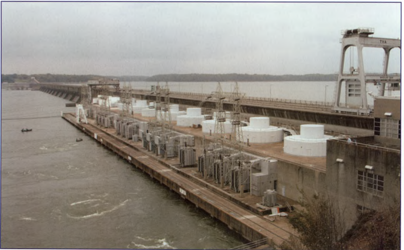
(Below) Wheeler Dam on the Tennessee River provides flood control and hydroelectric power.
