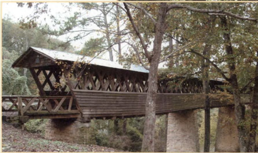
(Above) Covered bridges, like this one in Cullman County, were built throughout the state. The covering protected the bridge in bad weather.
