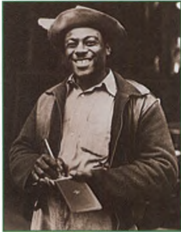
(Above) This man is a supervisor working on the construction of Wilson Dam (below) on the Tennessee River near Florence.
