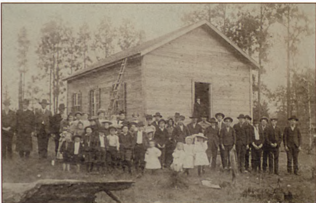
(Left) A newly built public school in Heflin, Alabama
