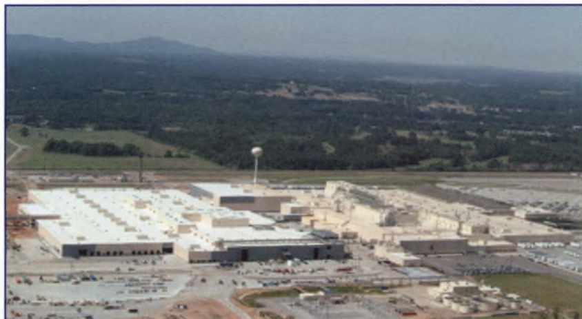
(Above) The new Honda automobile plant near Lincoln
