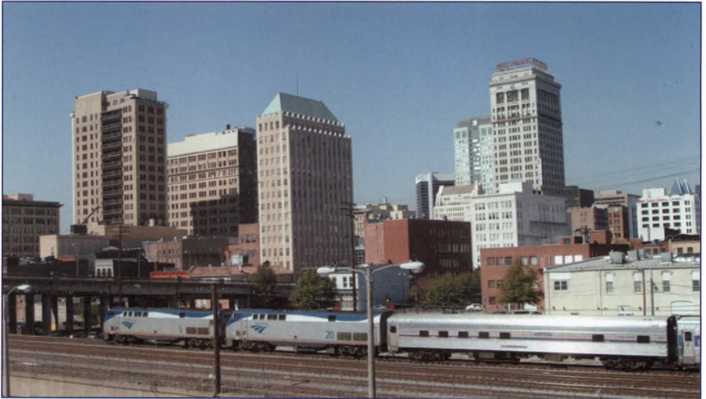
(Below) Birmingham's skyline shows a combination of old and new buildings.
