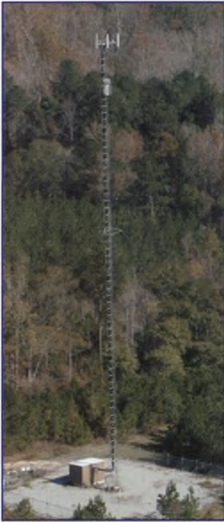
(Above) A communications tower
